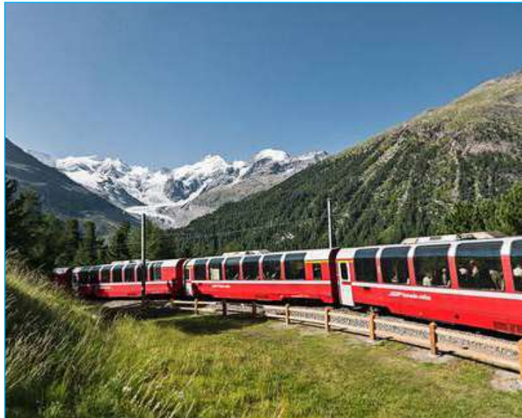
Fig. 18.3.5: Railway transport in Switzerland
