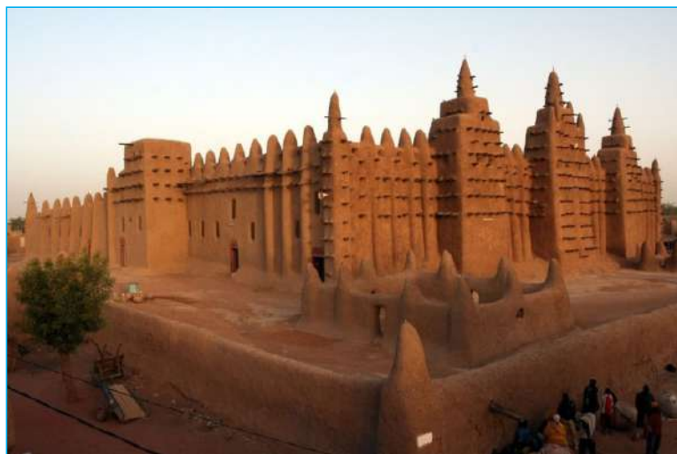
Fig. 17.3: The Great Mosque of Djenné in Mali
