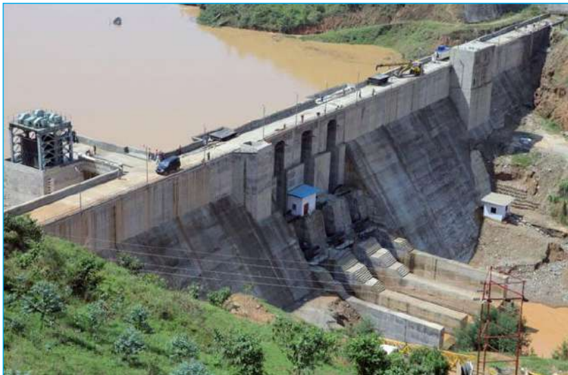
Fig. 14.2: A hydro-electric power station on River Nyabarongo
