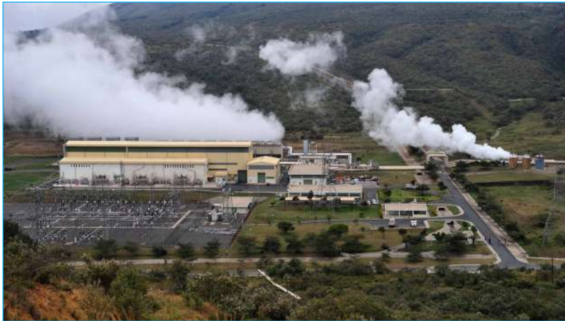
Fig. 14.3: Olkaria geothermal station in Kenya
