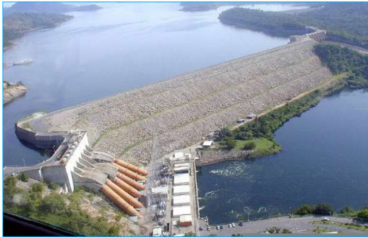
Fig. 14.7: Akosombo Dam on River Volta
