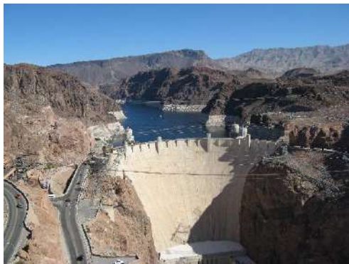
Fig. 18.2.3.3: Hoover Dam, USA
