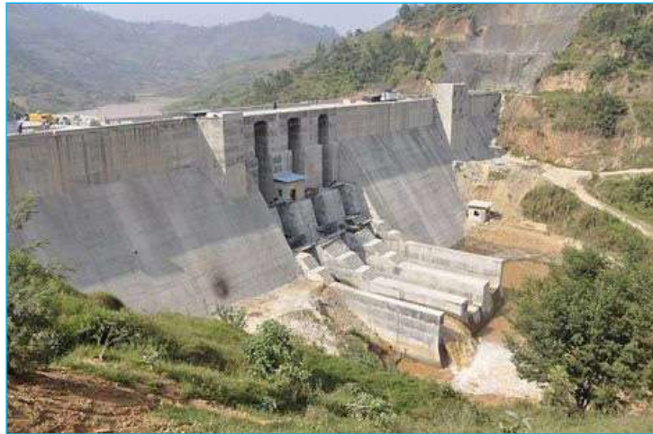
Fig. 6.5: H.E.P station on River Nyabarongo
